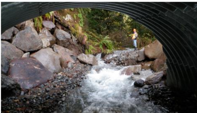
Large pipes with natural stream bottoms, called culverts, are used under roads in the watershed so that fish have access to their spawning streams.
